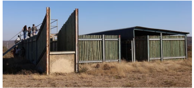
A buffalo boma developed through the DFFE Environmental Protection and Infrastructure Programme.
